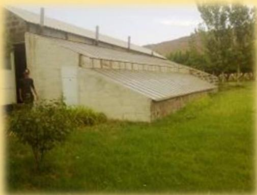
By combining electric and solar drying units, a technology change for dry fruit production was performed in “Ervandashat agricultural association” consumer cooperative company. As a result of using solar energy the saving of electricity amounted to around 75% or 4.7 MWh annually. Emissions reduction amounted to 2 tons of CO<sub>2</sub> eq. The annual saving is equal to 200 thnd AMD and the payback period is 10 months. There are evident environmental benefits.
