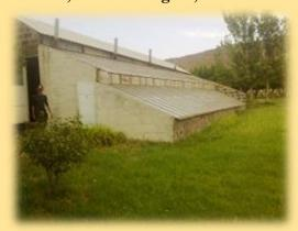
By combining electic and solar drying units, a technology change for dry fruit production was performed in "Ervandashat agricultural association" consumer cooperative company. As a result of using solar energy the saving of electricity amounted to around 75% or 4.7 MWh annually. Emissions reduction amounted to 2 tons of  $CO_{2 eq}$ . The annual saving is equal to 200 thnd AMD and the payback period is 10 months. There are evident environmental benefits.
